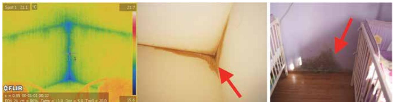
Figure 13. Thermogram of thermal bridge in the existing NZEB family house in Zagreb (left), consequences of thermal bridges (centre and right)
