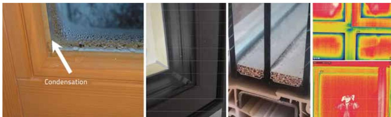
Figure 16. Condensation of water vapour at the glass edge (left), composite and aluminium glass edges (centre), thermogram of thermal bridge at glass edge (right)
