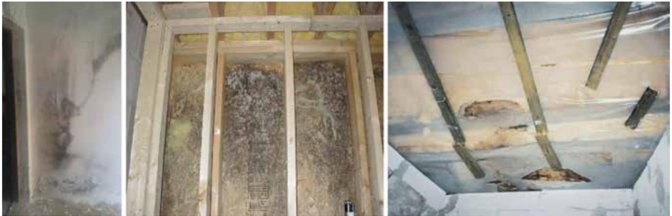
Figure 7. Funghi and mould growth on the surface (left) and within building elements (centre and right)
